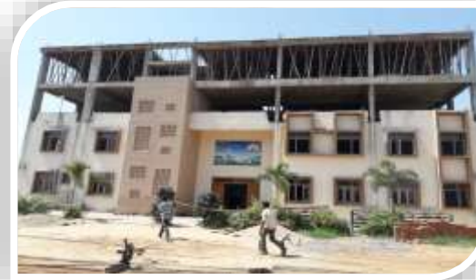
Provided AAC Blocks to construct floor to govt. School
