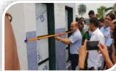
Construction of public Toilet at Nare village near Wada plant
