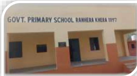
Renovation of Primary Govt School at Faridabad
