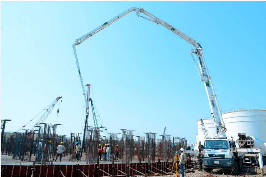
Precast Piling at Kandla
