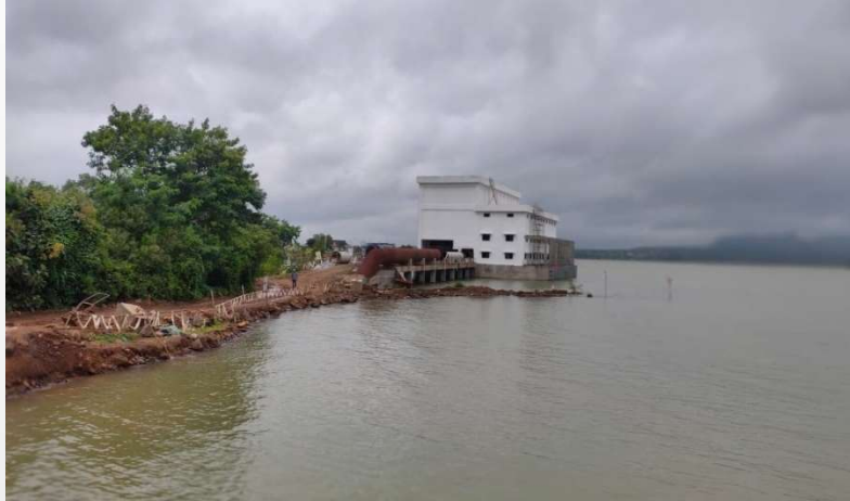
Bhama Askhed Water Supply Project
