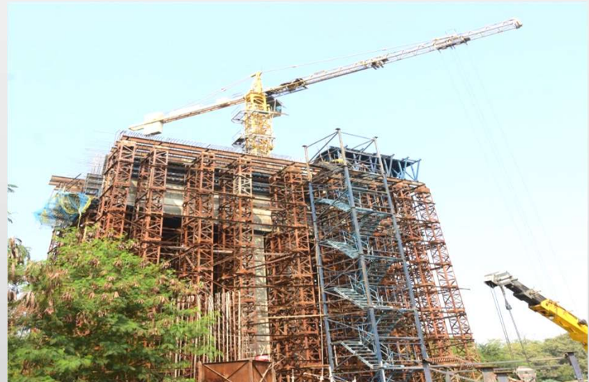
Nagpur Metro Station – Under Construction
