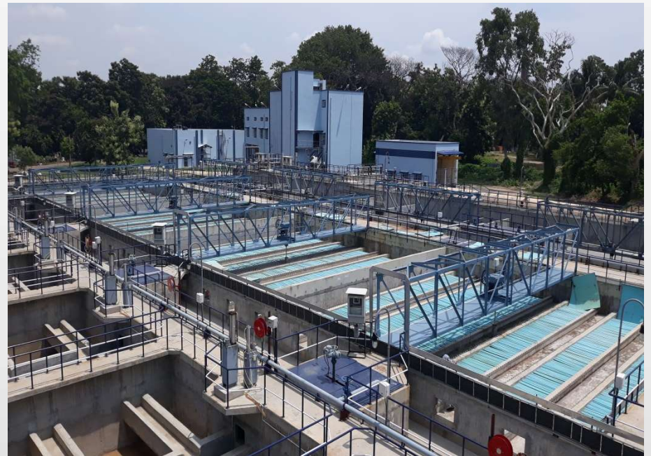
Palta Water Works - WTP
