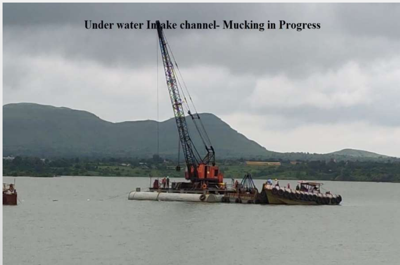
Irrigation Work in progress, Bhama, Pune
