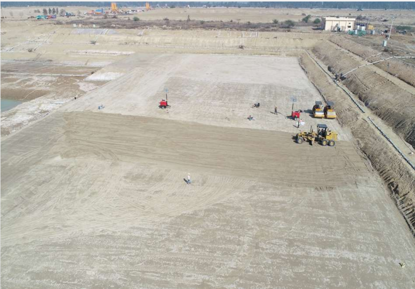
Ground Improvement Nuclear Power Project
