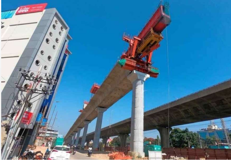
Bangalore Metro Segment Erection
