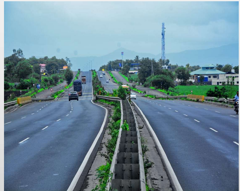
Pune Satara Road Project
