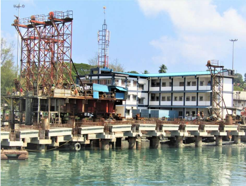
Jetty under Construction, Andaman
