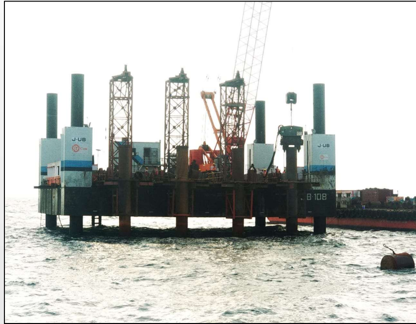
Construction of Permanent Piles by Jack up at Udangudi Project
