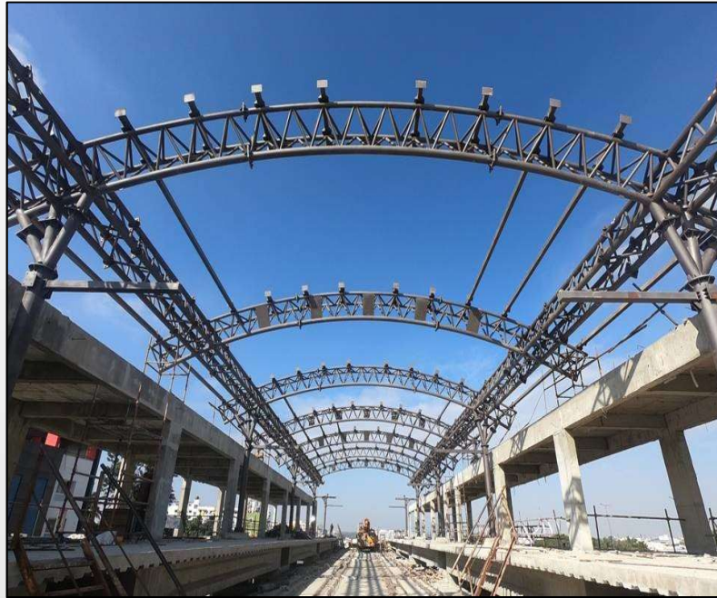
Bangalore Metro RK Puram Station Construction
