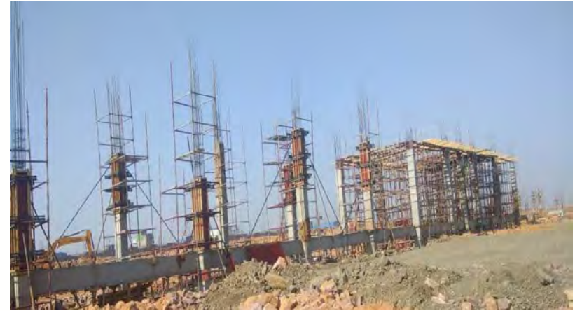
Engine line building
