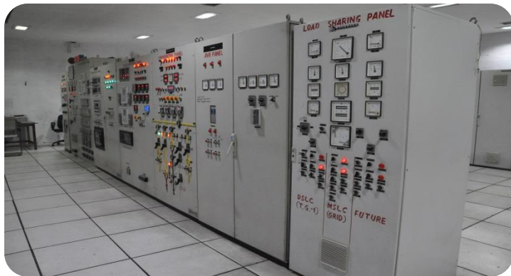
Cogeneration Control Panel
