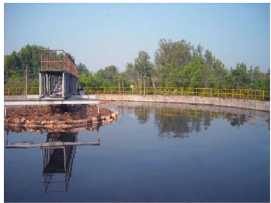
Primary Clarifier - Paper
