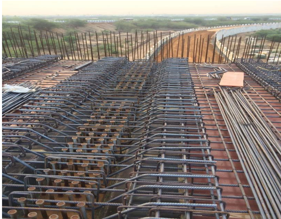
Flyover in Madurai - Ramanathpuram Section
