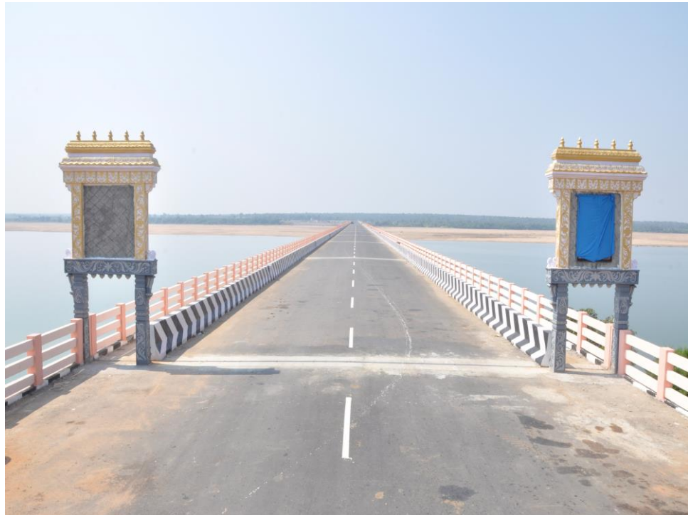
Eturunagaram Bridge over river Godavari
