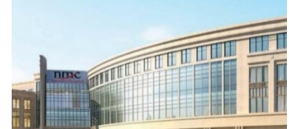
NMC Speciality hospital, Abu Dhabi
