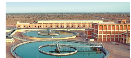
Water Treatment Plant, Barmer
