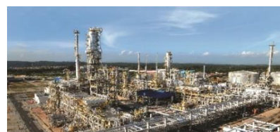
Petronas Refinery, Malaysia
