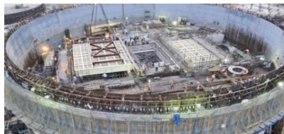
Kakrapar Nuclear Power Plant, Guj
