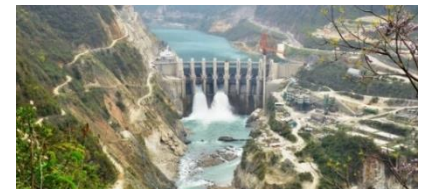
Srinagar Hydro Electric Plant
