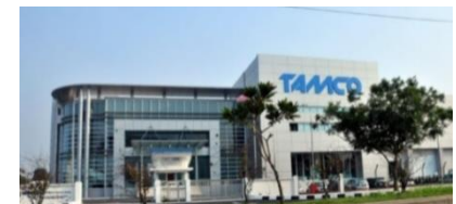
MV Switchgear Factory, Malaysia
