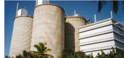
Bulk Cement Terminal, Colombo
