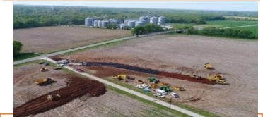
Broke ground May 2018 Guthrie, Kentucky
