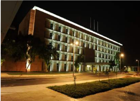
Swarnim Sankul 1 & 2 Construction and interior work
