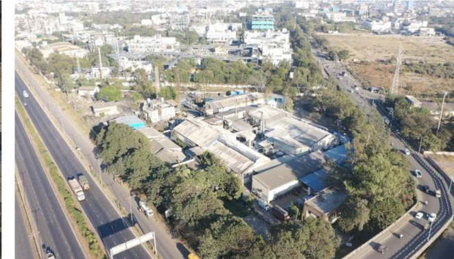
Our Ankleshwar Facility - Gujarat
