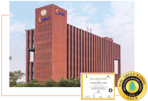
Max House - Certified LEED Gold certified and Health and Wellbeing Gold from IGBC
