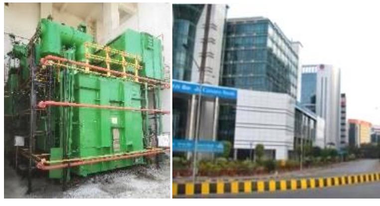
Ester-filled transformer commissioned for Tata Power – delivering environmental value
