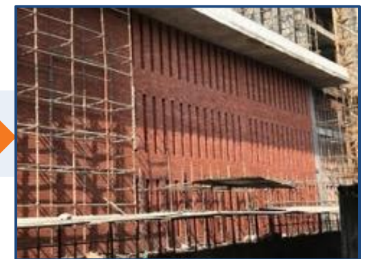
September 2019 Structure completed
