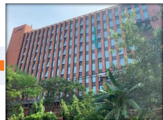
June 2020 Glass Façade Completed
