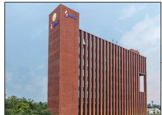
August 2020 Construction Completed
