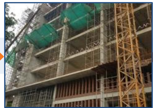
June 2019 Structure completed upto L6
