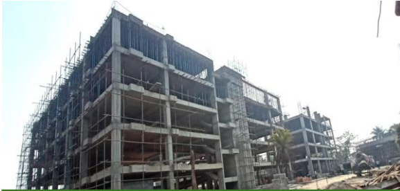
Medical and healthcare facility under construction
