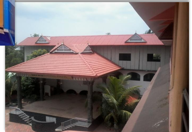
Roof Top Extension - (V-Panel )
