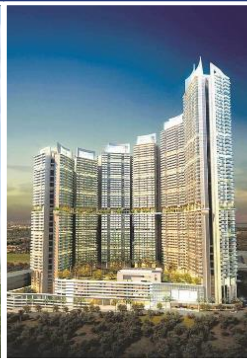
L&T Crescent Bay
