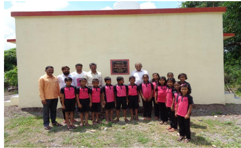
Constructed Ladies And Gents Toile Block At Innovative School Ankoli Tal Mohol Dist Solapur Dt 03.09.2022
