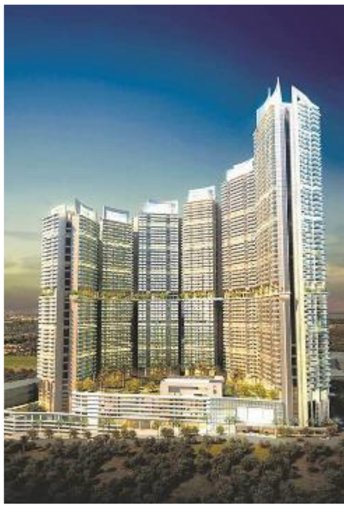
L&T Crescent Bay
