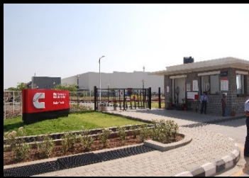
HHP Rebuild Center 2011
