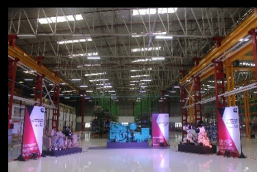
Power Systems Plant , Pirangut 2018
