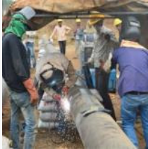
Thumbli Water Pipeline– Cairn Energy India – Rajasthan
