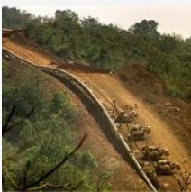
Panvel Dabhol Pipeline Project–Gail Ltd - Maharashtra
