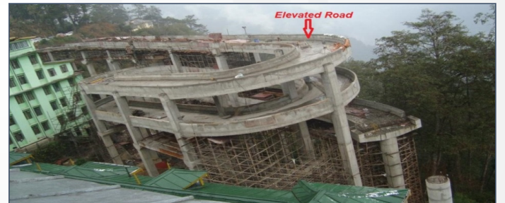
Piling & Civil Arctech, Gangtok
