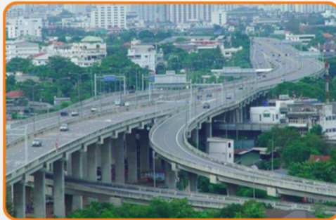
Ramindra - At Narong Expressway System
