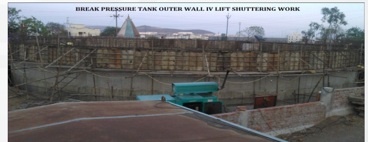
Break pressure tank work in progress, Bhamra, Pune
