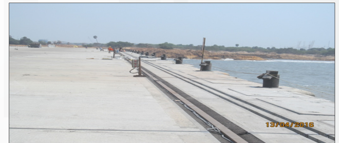
Ennore container terminal, Chennai
