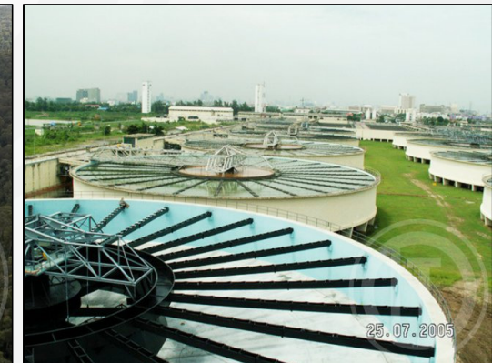
Bang Khen Water Treatment Plant , Bangkok
