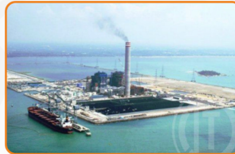
BLCP 2 x 700 Mw Coal Fired Power Plant (Civil Works)
