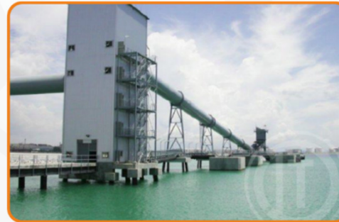
COCO Coal Handling System
