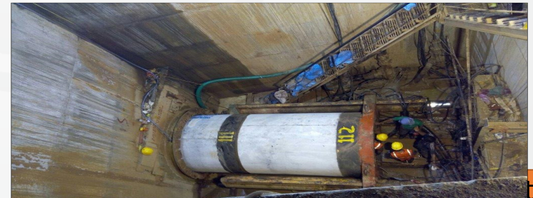
VMSS – Micro Tunneling Vadodara
