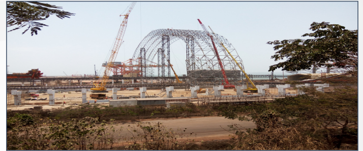
JSW Jaigad counterfort columns
