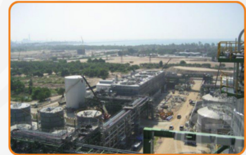
Piping works for PTT phenol project
