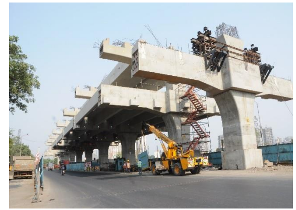
Mumbai Metro Line 6
