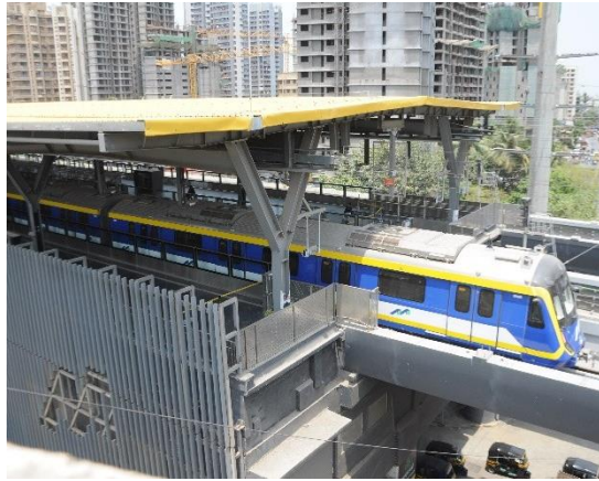
Mumbai Metro Line 2A
