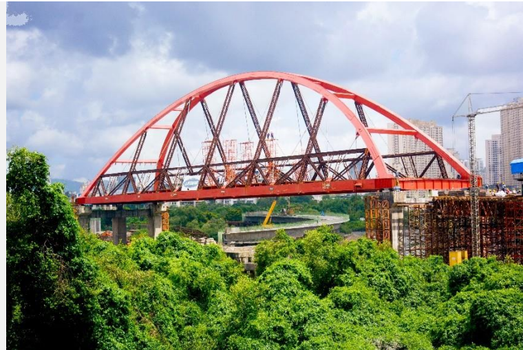
Kalwa Bridge Thane
