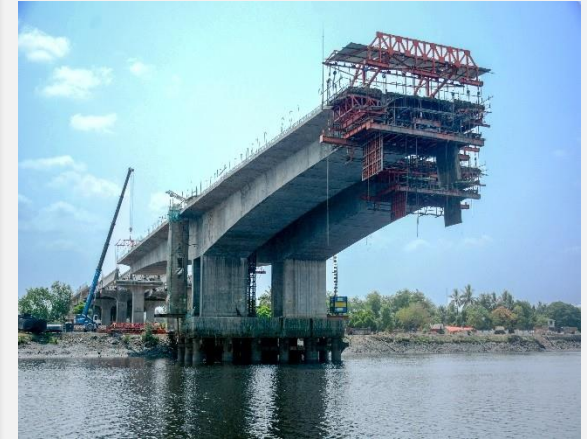
Motagaon Creek Bridge
