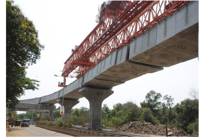
Airoli Creek Bridge
