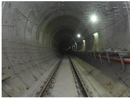
Mumbai Underground Metro Line 3
