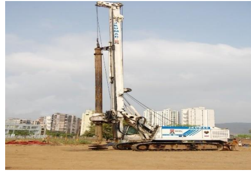
Hydraulic Piling Rig
