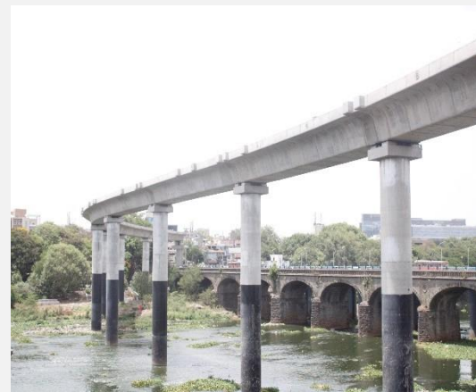
Pune Elevated Metro
