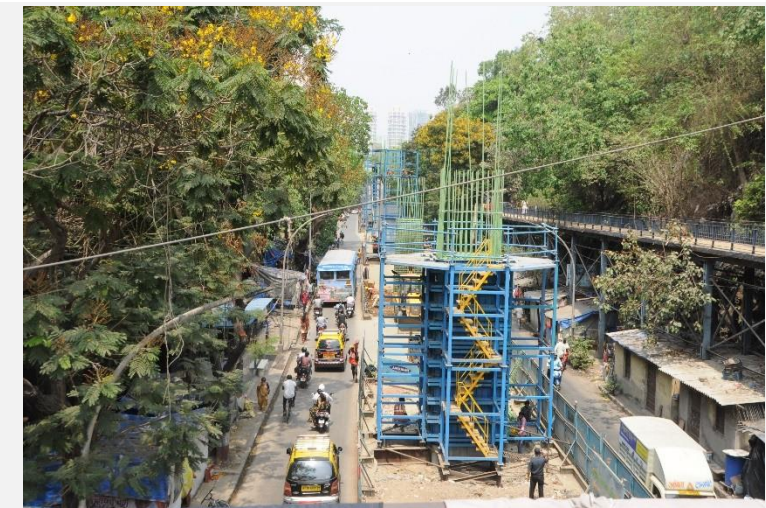
Sewri Worli Elevated
