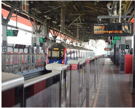
Mumbai Metro Line 7
