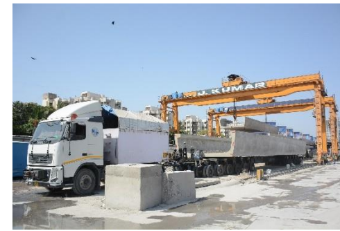
Casting Yard - Elevated Metro
