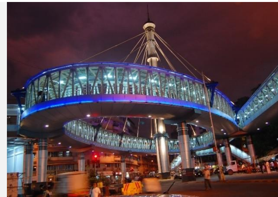
Grant road Skywalk
