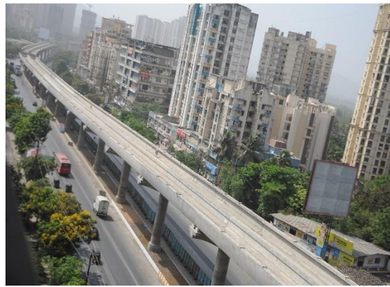
Mumbai Metro Line 4A
