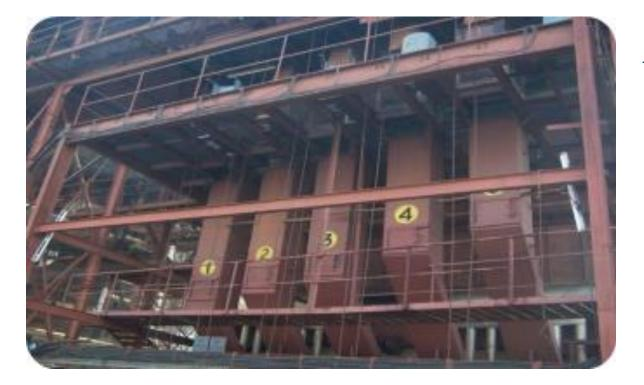
Bagasse Silos & Feeders of Boiler
