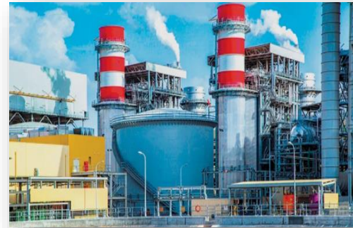
1,516 MW IBRI IPP, SEPCO – 3, Oman (Completed Project)
