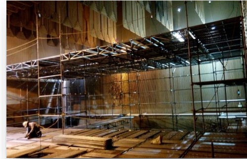
Cuplock Scaffolding Erection 800 MW, Mundra
