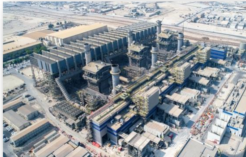
1,800 MW Alba PS5 CCPP, Bahrain (Completed Project)
