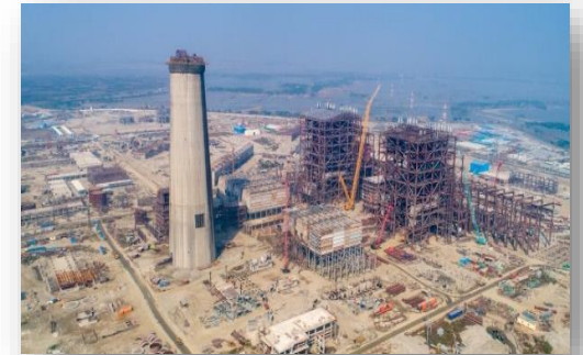
2X660 MW at Rampal, Maitree, Bangladesh-BIFPCL
