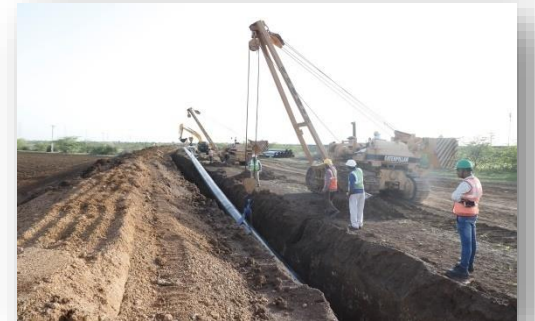
Lowering of Pipe Section, Mundra, Adani
