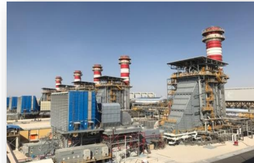
1,519 MW Fadhili CHPP, Doosan, KSA
