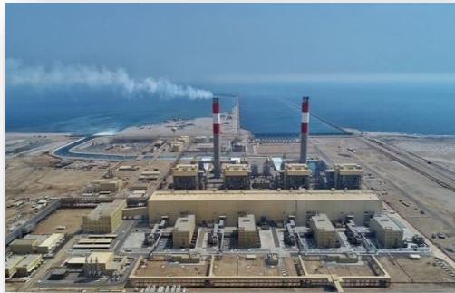
4X660 MW Shuqiaq SSPP, KSA (Completed Project)
