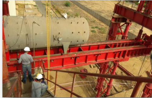
HP Heater Replacement 800 MW, CGPL Mundra 2
