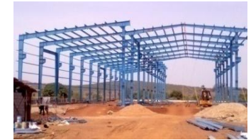
Pre Engineering Building
