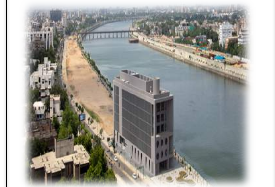
Sabarmati Riverfront Development Co. Ltd. (SRFDCL) Office Building, Ahmedabad
