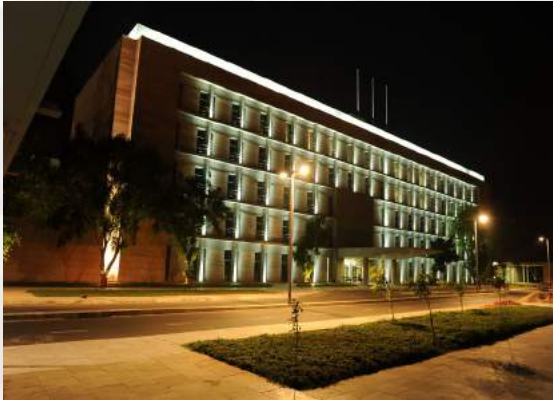
Swarnim Sankul 1 & 2 Construction and interior work
