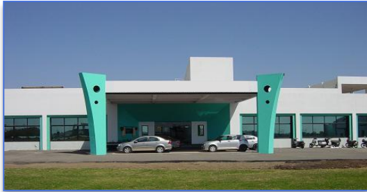
Dedicated R&D facilities at Rajkot and Strasbourg
