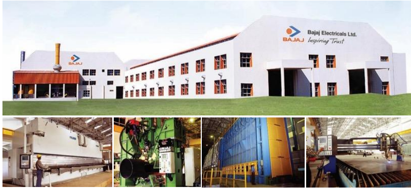
Poles & High-mast factory at Ranjangaon, Pune, India
