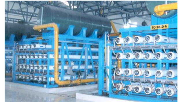
DEMINERALIZATION PLANTS FOR THERMAL POWER STATION
