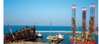
Fabrication Facility, Oman
