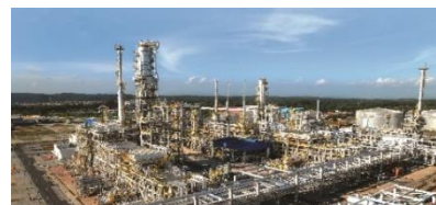
Petronas Refinery, Malaysia
