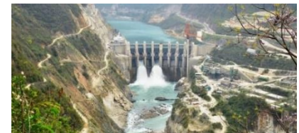
Srinagar Hydro Electric Plant
