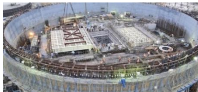
Kakrapar Nuclear Power Plant, Guj
