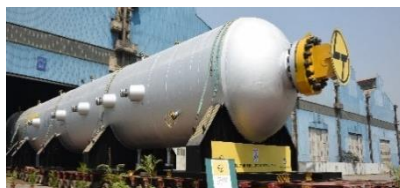
Hydrocracker, HPCL Visakh Refinery
