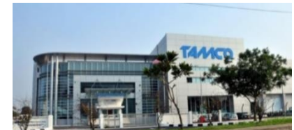
MV Switchgear Factory, Malaysia
