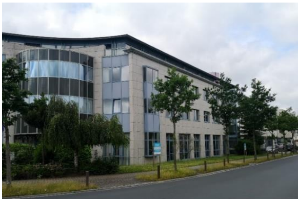
R&D Office, Germany
