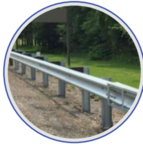
Metal Beam Crash Barrier
