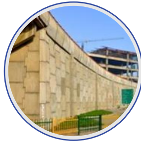
Reinforced Earth Walls
