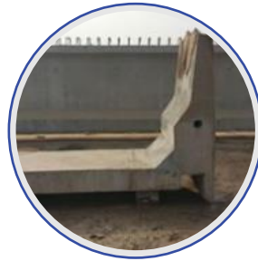
Fabricated Casting Panels and Moulds
