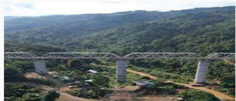
Construction of foundation and sub structure over pile foundation for Tall Bridge of new BG Railway line from Bairabi to Sairang (Mizoram).
