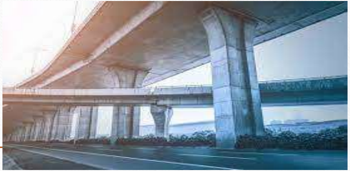
Maintenance of 3 lane Brahmaputra Bridge including their expansion joints & bearing, providing all necessary signboard, road furniture etc..
