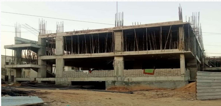
Construction of Pediatrics Block and multi level parking.
