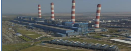
Erection, Testing & Commissioning - BTG & BOP
