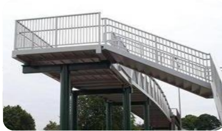
Stainless steel Foot-over-bridges
