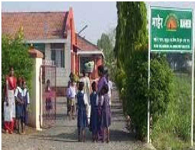
Maher Renovation of 8 toilets + 2 girls rooms - @ Vadhu
