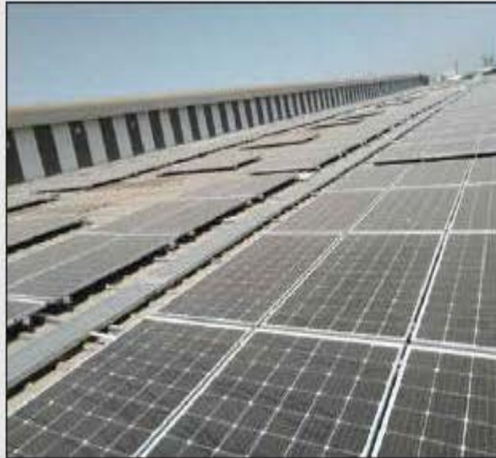
Installation of Solar panels
