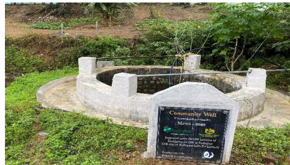
Well Restoration – Kalvarayan * Jawadhu Hills
