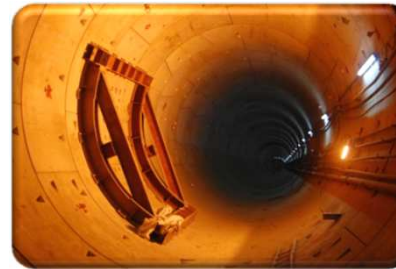
DMRC CC-24 Tunnel
