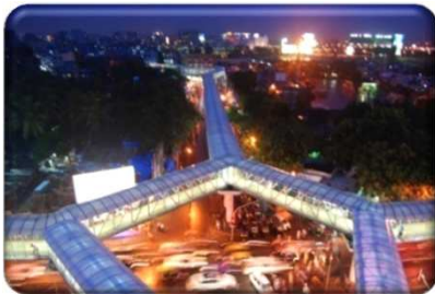
Skywalk at Bandra, Mumbai
