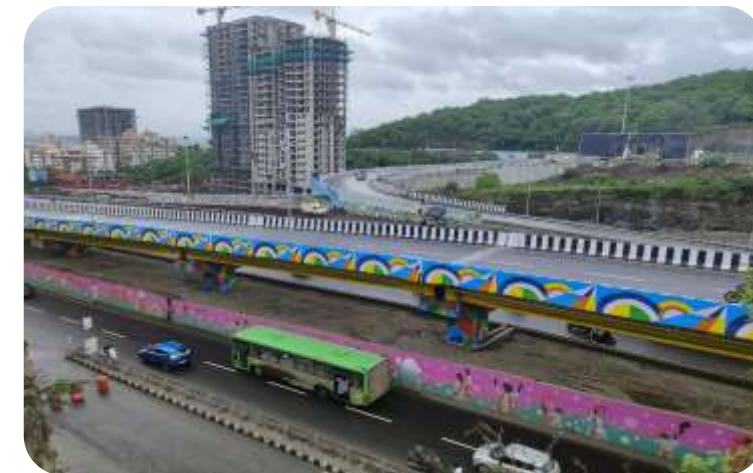
Chandni Chowk Flyover, Pune
