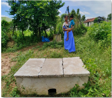
Waste management through bio-digesters, using the cattle waste to provide biogas to rural homes.
