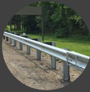
Metal Beam Crash Barrier
