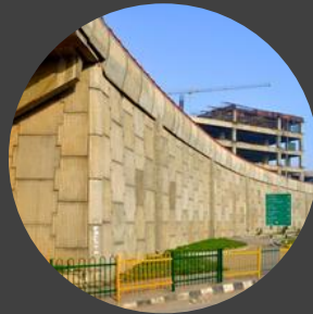
Reinforced Earth Walls
