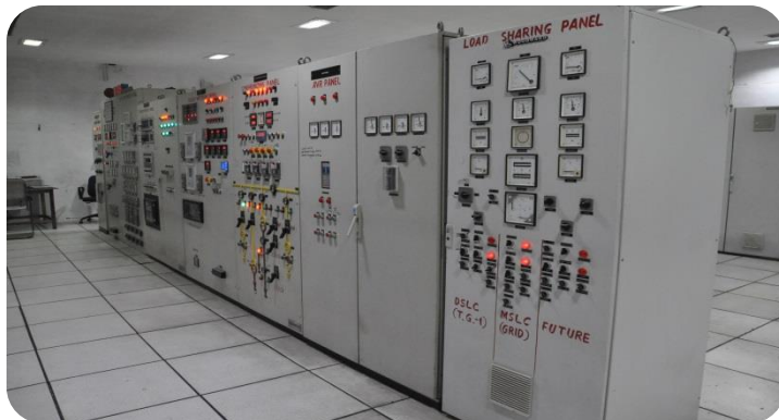
Cogeneration Control Panel
