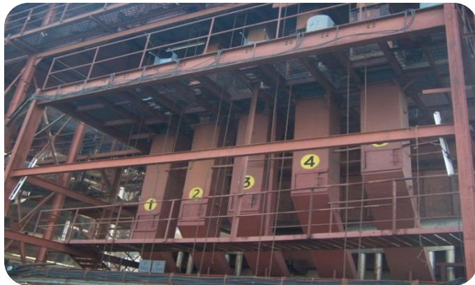
Bagasse Silos & Feeders of Boiler
