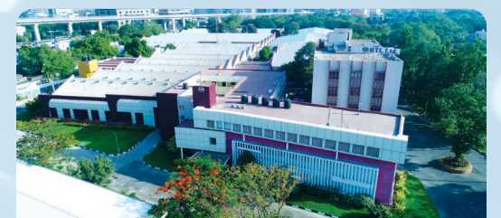
Chennai, Tamil Nadu (through subsidiary company HTL Ltd) 3
