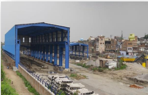
MEMU Shed at Kanpur-RVNL
