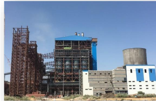
2x660 MW Suratgarh STPP, RRVUNL
