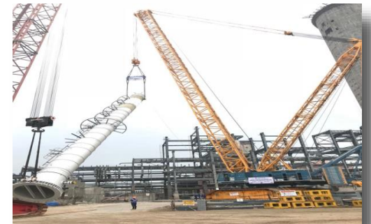
Urea Reactor Tank Installation At Ramagaundam, Telangana
