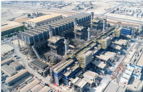
1,800 MW Alba PS5 CCPP, Bahrain (Completed Project)
