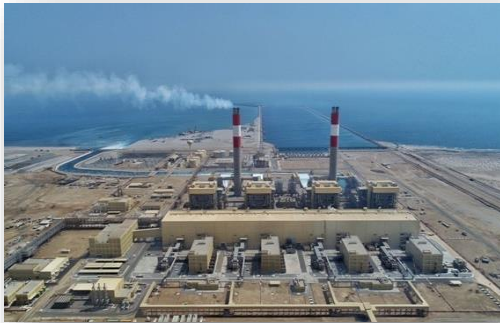
4X660 MW Shuqiaq SSPP, KSA (Completed Project)
