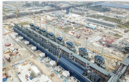
400 MW Dangote Oil Refinery & Petrochemicals Project, DORC, Nigeria
