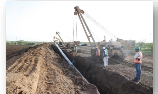
Lowering of Pipe Section, Mundra, Adani
