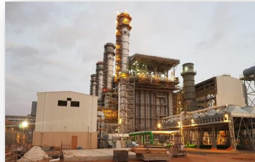
1,390 MW Waad Al Shamal ISCCPP, GE, KSA
