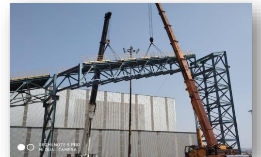
Erection of P&N Gallery at Bellary, JSW
