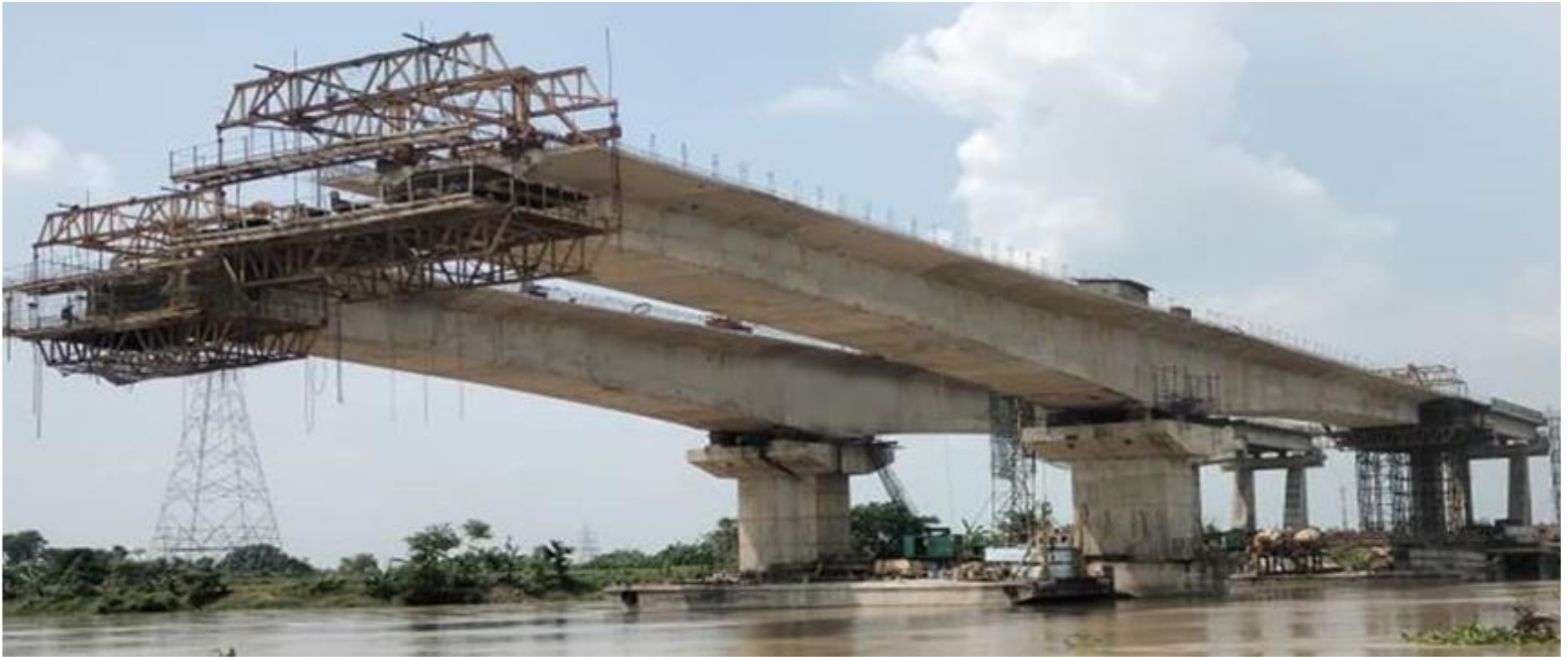
Bhagirathi bridge super structure works at Baharampore Bypass
