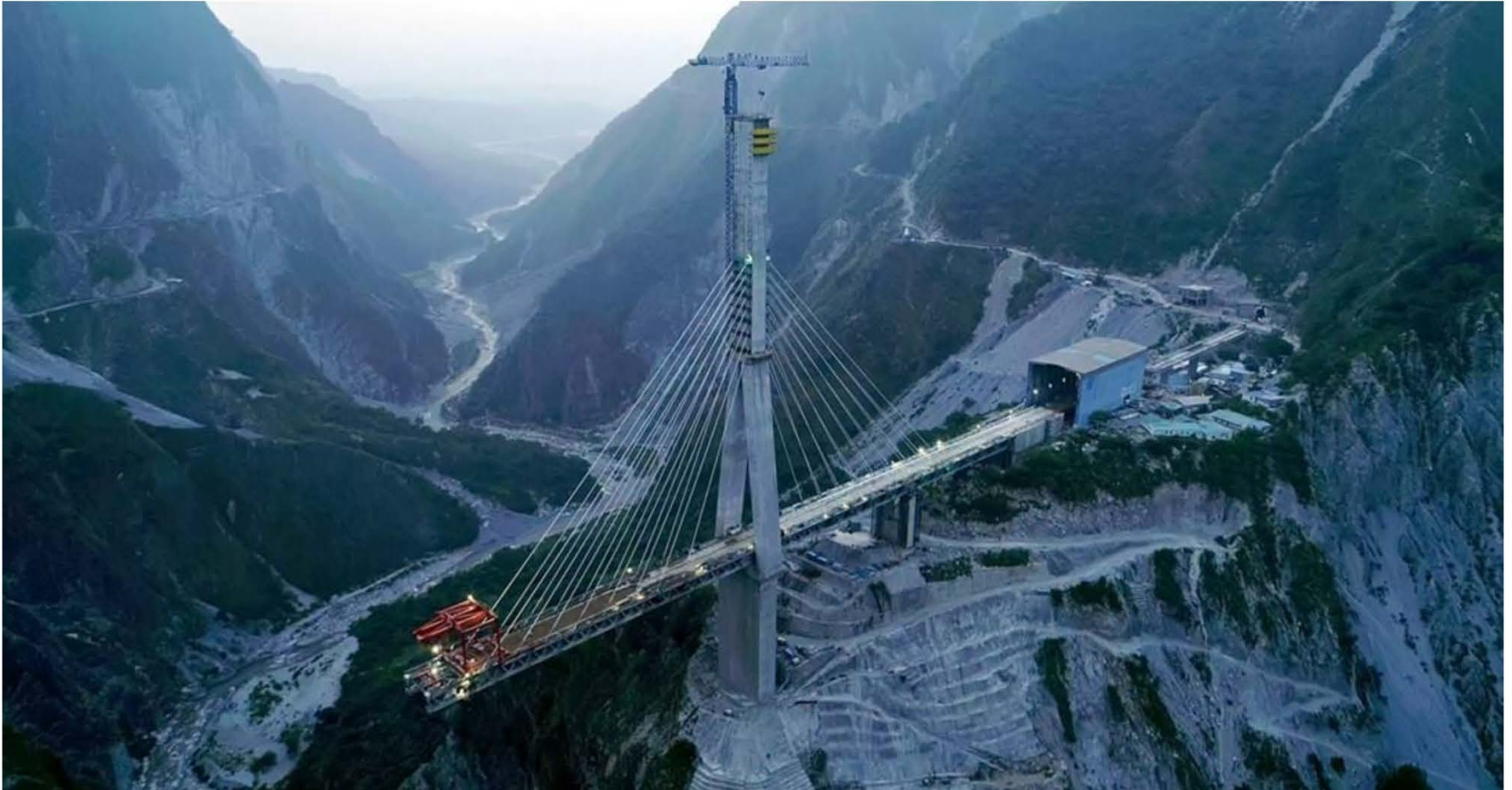
Segments launching in progress
