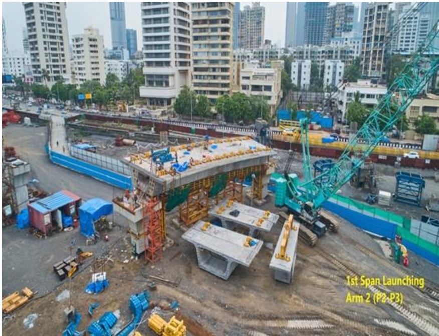
Arm-2 - Segment Launching of 1 st Span
