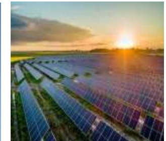
Solar Mounting Structures
