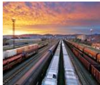
Dedicated Fright Corridor
