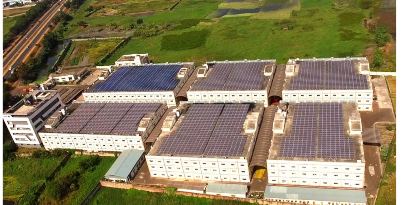
Rooftop solar power plant at Dankuni unit
