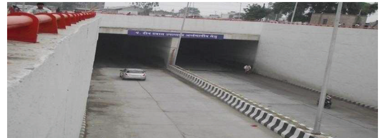
Construction of RUB at Badli, New Delhi
