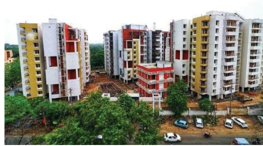
Construction of 222 Flats at Keelandev Tower, Bhopal for MP Housing & Infrastructure Development Board
