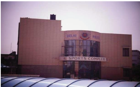
Police Station & Residential Quarters at Kondli, New Delhi for MHA, Delhi Police through RITES Ltd.
