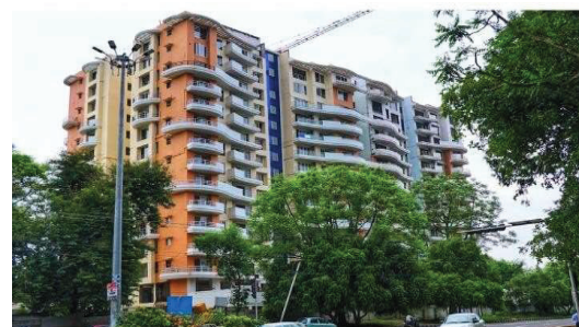
Construction of 96 flats at Tulsi Tower, Bhopal for MP Housing & Infrastructure Development Board
