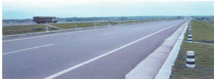
Maintenance of NH-19, (earlier NH-2) Barwa Adda – Panagarh Section (KM 398.75 – KM 512.00) in the state of Jharkhand & West Bengal
