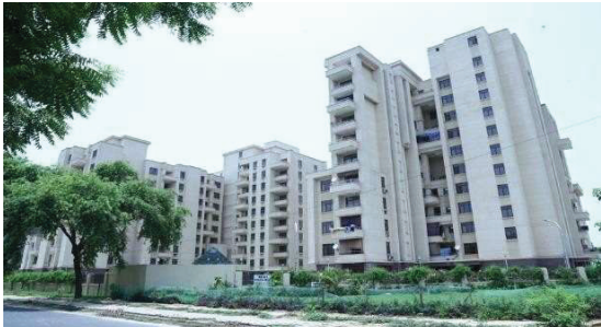
Residential accommodation for NHA staff at Sector 17, Dwarka, New Delhi
