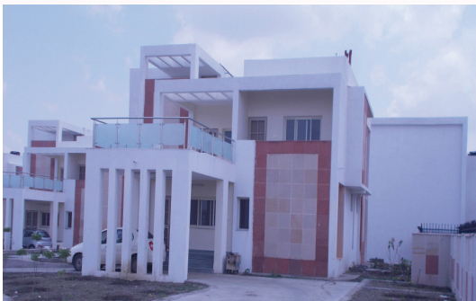
Construction of Director, Dean Bungalow, QIP Centre & Accommodation for School of Planning & Architecture at Bhopal
