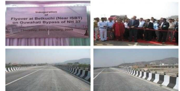
Construction of 2 lane flyover on Guwahati Bypass of NH-115 (earlier NH-37) in the state of Assam
