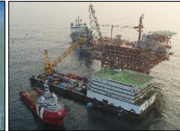
Construction Works at Control Riser Platform
