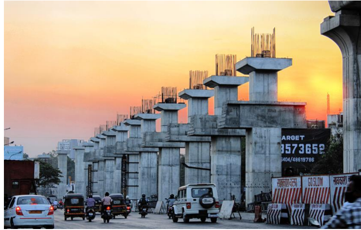
Pune Elevated Metro
