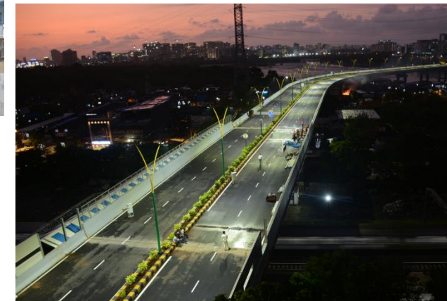
BKC- Chunabhatti Flyover
