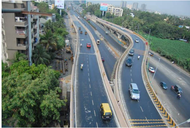
Amar Mahal Flyover
