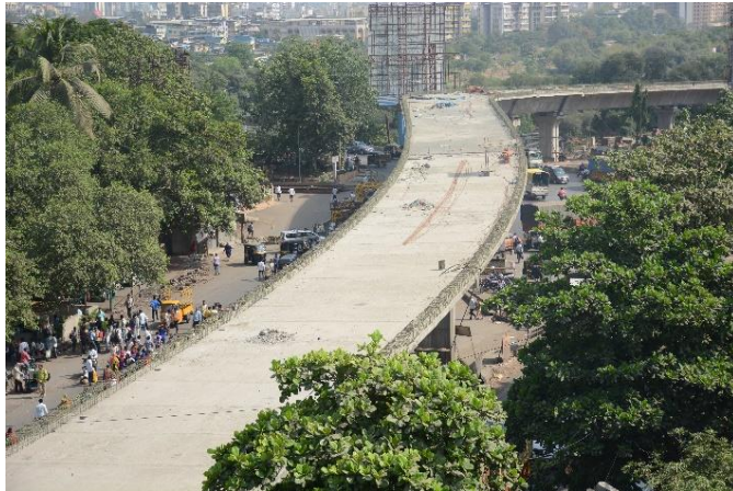
Kalwa Bridge Thane
